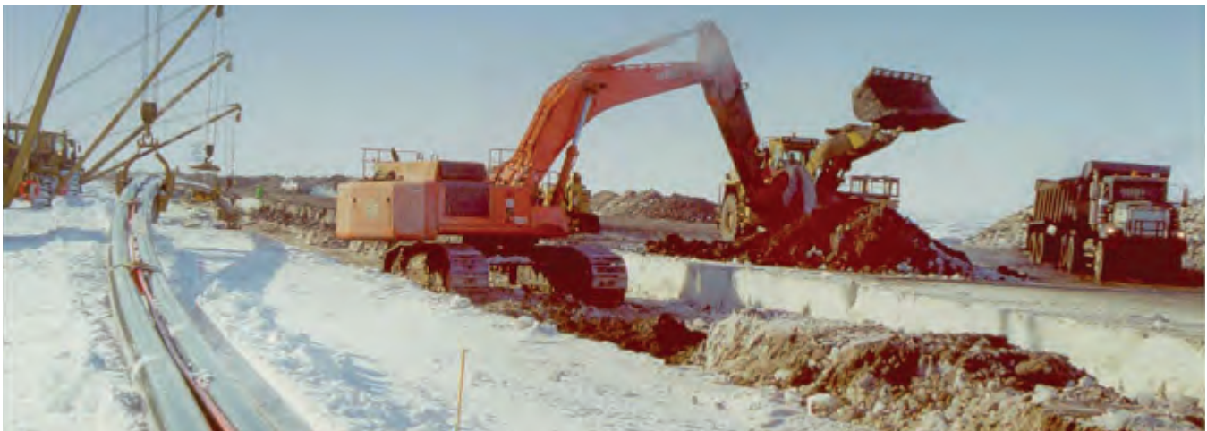
Figure 2-13. Construction of Northstar Offshore Pipeline
