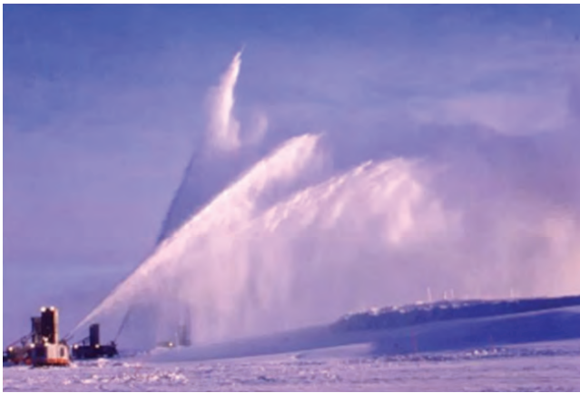
Figure 1-31. Spray Ice Island Construction
