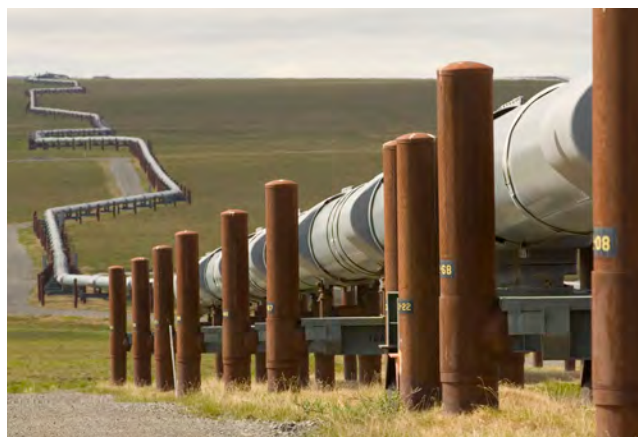
Figure 1-26. Trans-Alaska Pipeline Zigzag Design
