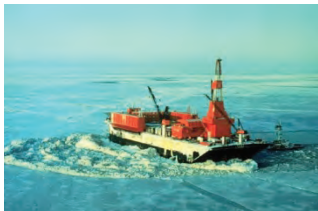
Figure 6-19. Example Ice Damage Zone at the SSDC Platform in the Beaufort Sea
